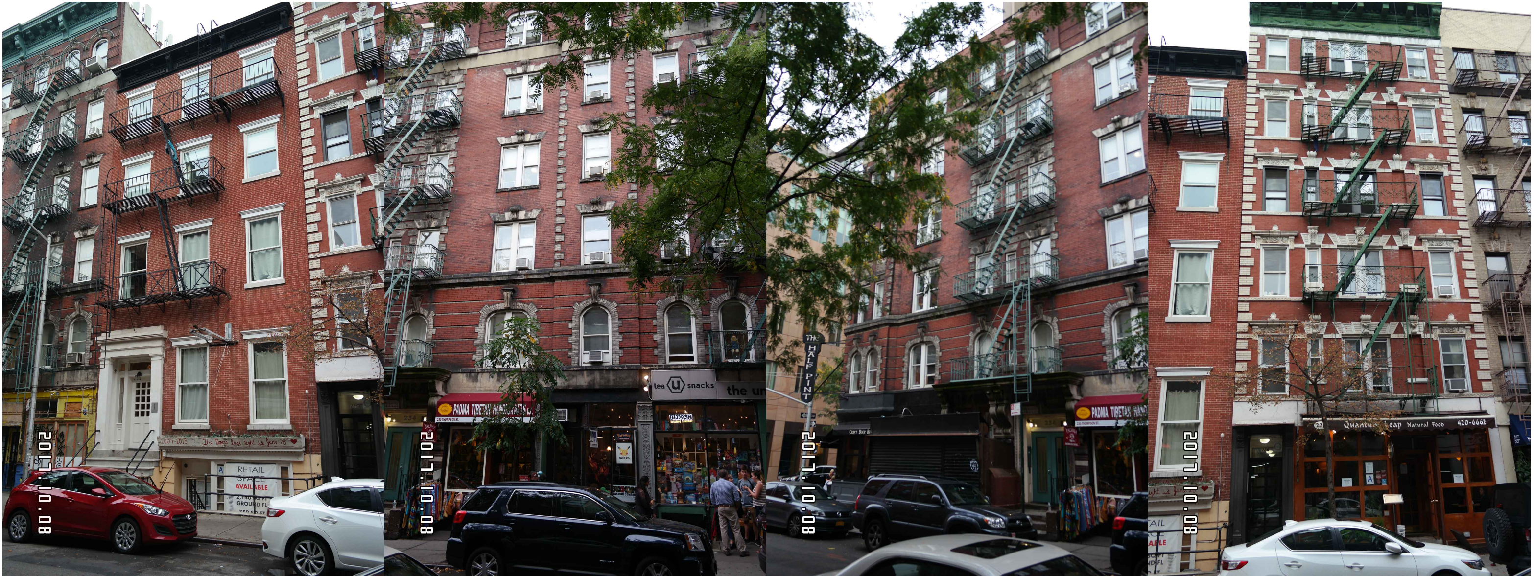
© ADJACENT BUILDING ON THOMPSON STREET
